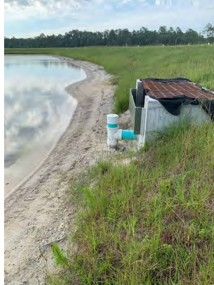
Pond control structure – Phase 5
