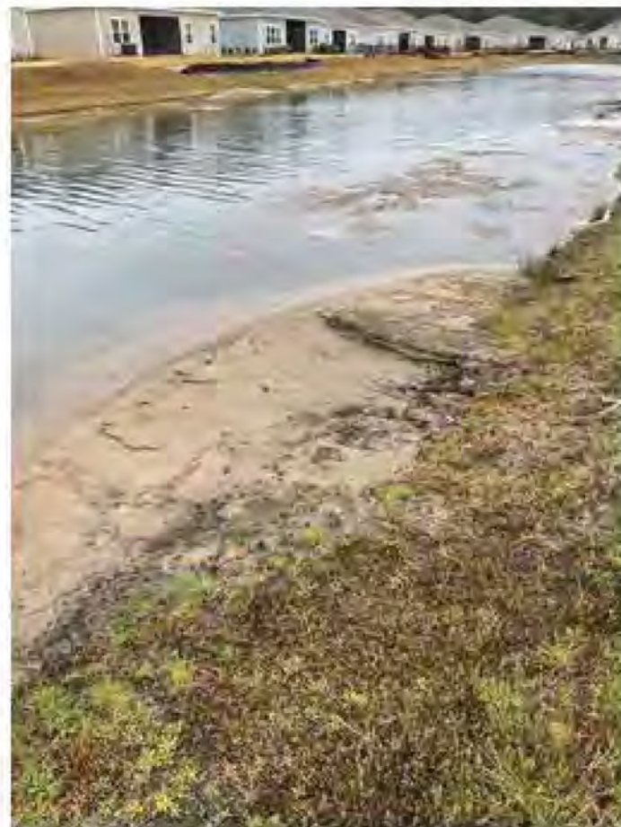
Erosion of Pond Bank Phase 4 (Pond 14)
