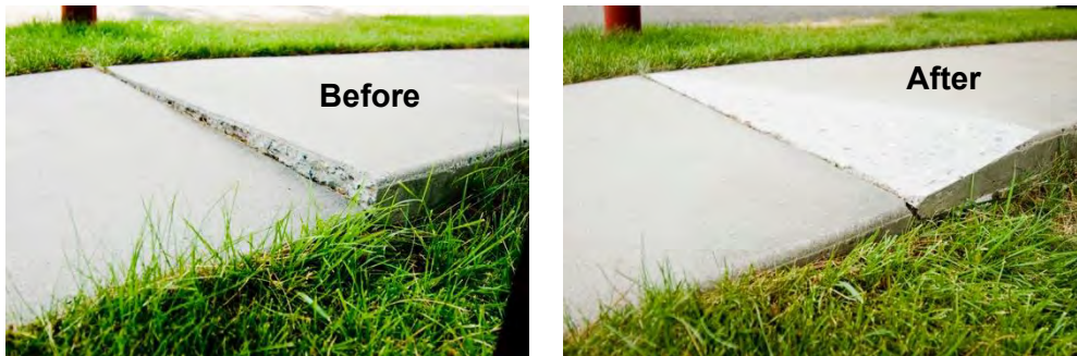
Figure 12: Precision Sidewalk Safety Work Example
