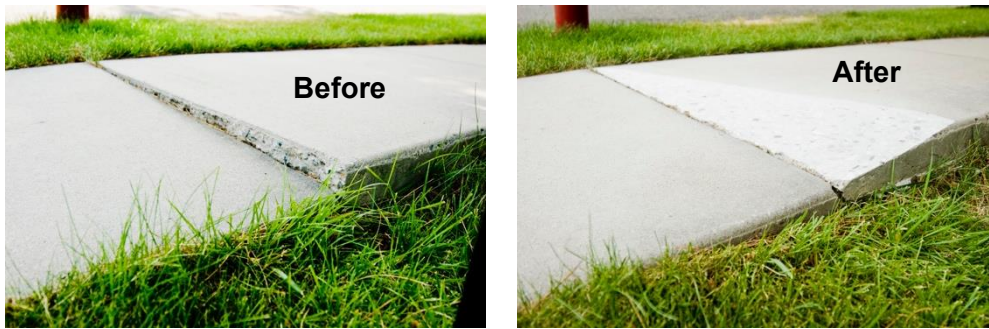
Figure 1 Precision Sidewalk Safety Work Example
