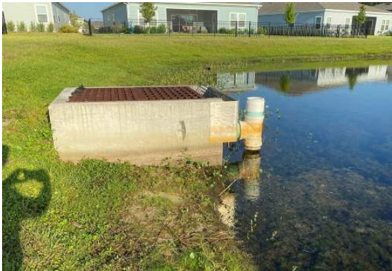
Inlet protection installed on phase 5b pond
