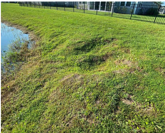
Erosion on phase 4B pond slope
