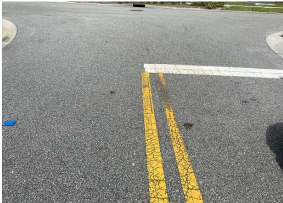
Faded striping in phase 2
