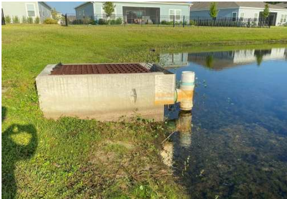
Inlet protection installed on phase 5b pond
