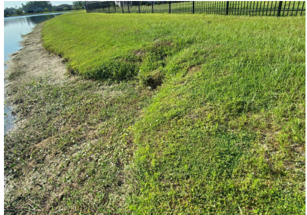
Erosion on phase 4A pond slope
