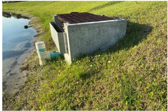
Inlet protection installed on phase 5b pond...also clean out under bottom of orifice pipe
