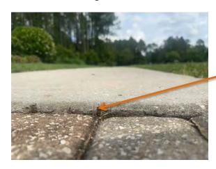
Example of a %" high "Severe" hazard located on a panel adjacent to a driveway composed of brick pavers that are not grouted into place on Majestic Walk Circle. As directed by the community, these types of hazards are included in this proposal.
