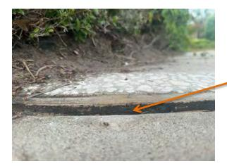
Example of a "Severe" hazard on Majestic Walk Blvd next to a wooden spacer. The concrete hazard will be repaired by PSSC however Amelia Walk should make arrangements to remove or cut the wooden expansion joint, which is raised along with the concrete as this is not a service PSSC provides.
