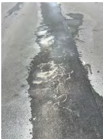
Evidence of high groundwater damaging asphalt
