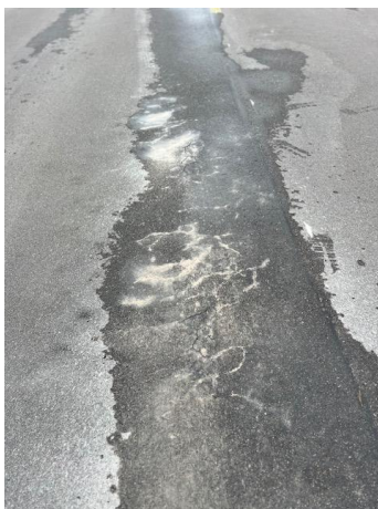
Evidence of high groundwater damaging asphalt
