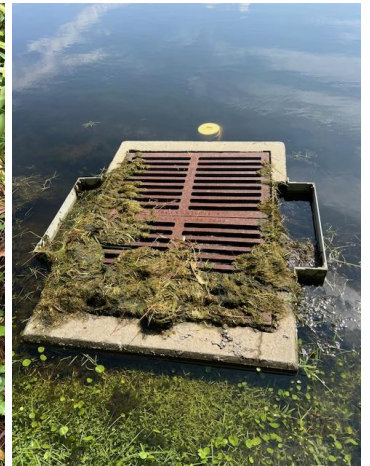
Debris covering Control Structure
