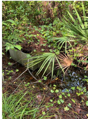
Debris covering Spreader Structure
