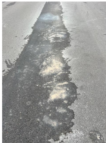
Evidence of high groundwater damaging asphalt
