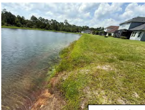
Pond bank erosion on Fallen Leaf Drive
