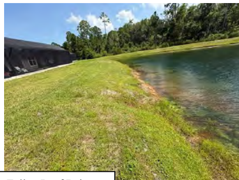
Pond bank erosion on Fallen Leaf Drive
