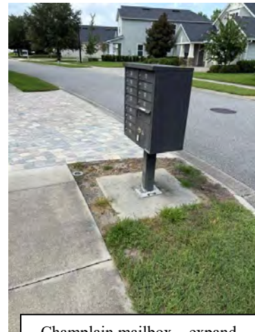
Champlain mailbox – expand concrete to meet sidewalk?
