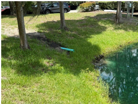
New drainage near clubhouse
