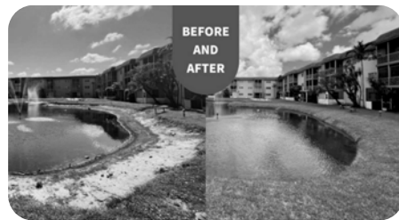
Erosion Repair & Prevention
