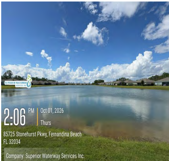
Pond 16 – Looks ok at this time.
